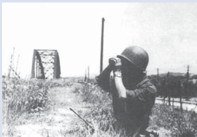
A soldier on watch from the South of the Han River (June 28, 1950) Following the destruction of the Han River Bridge, the South's troops that were isolated in north of the Han River, were reorganized and kept a defensive line south of the Han River until July 3, 1950.
